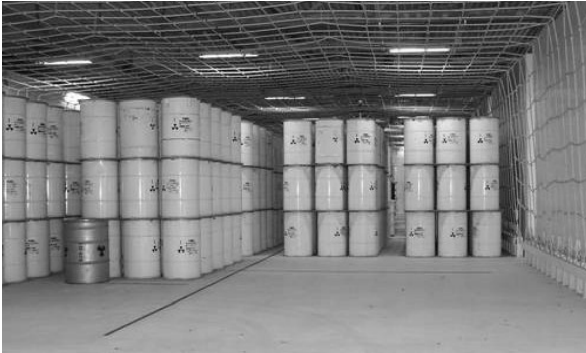
Figure 3: Caorso – ERSBA 2 storage facility
