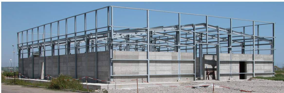
Figure 6: ITREC – The new storage facility under construction
