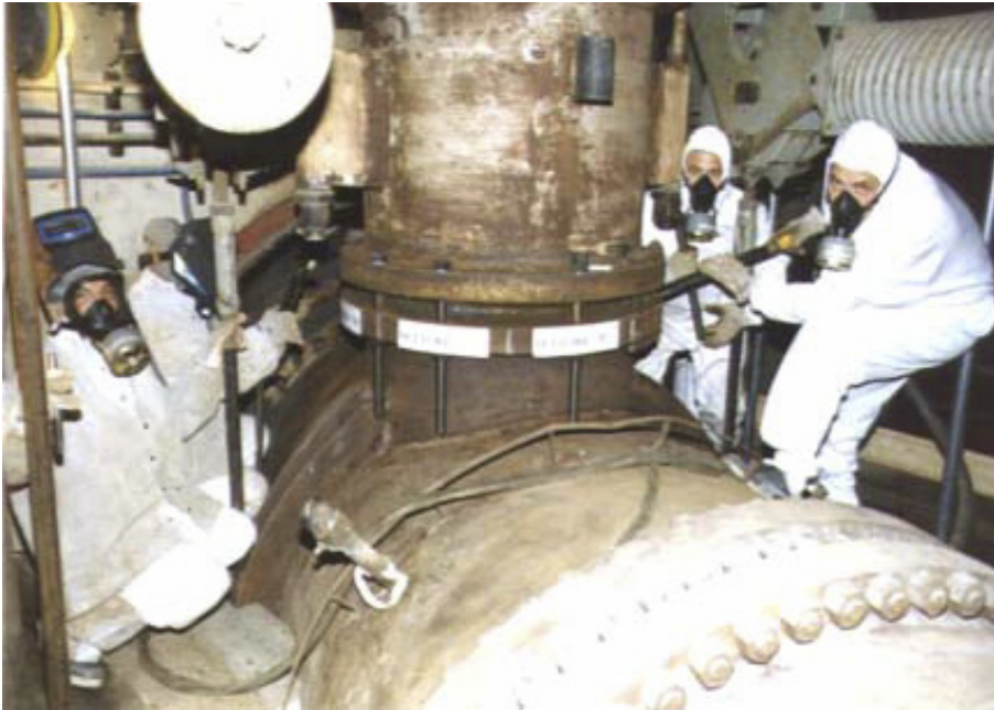
Figure 4: Latina NPP – preliminary dismantling activity of the primary circuit
