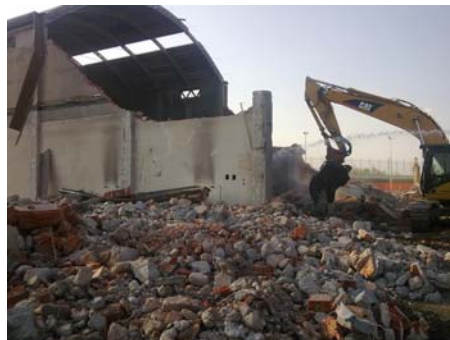
Eurex – Building 1600 Demolition
