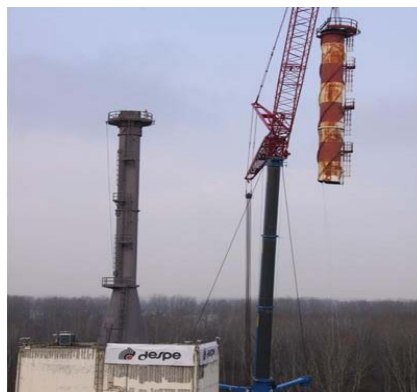
Caorso - Off-gas building - Stack removal
