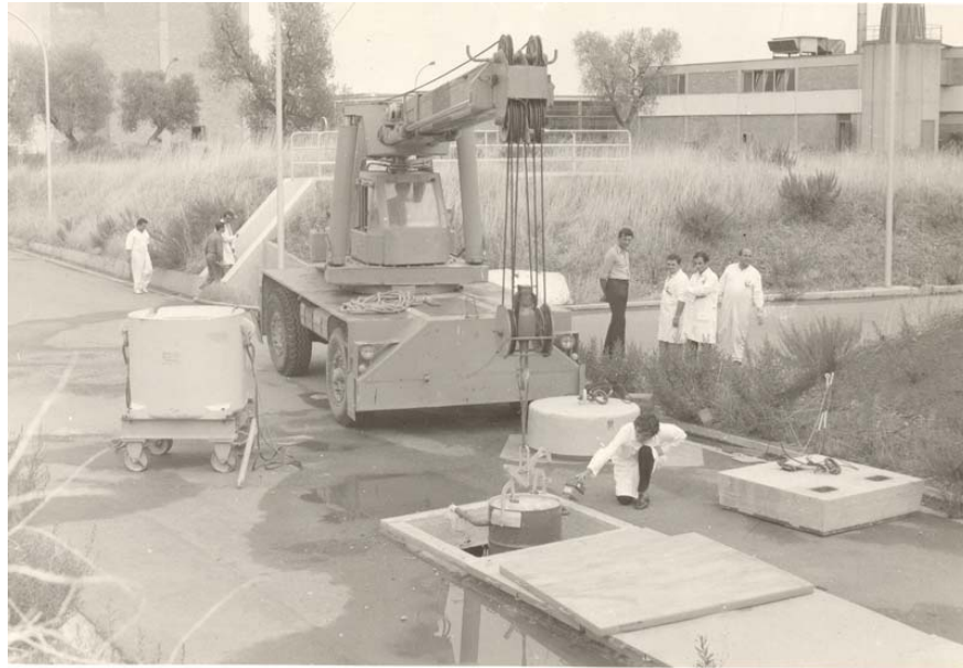
Figure 7: Historical picture of burial of radioactive waste in pits at the ITREC facility in the years '70s.
