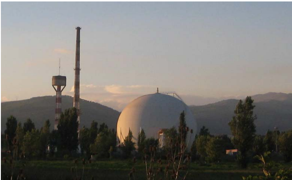
Figure 8: The chimney of the Garigliano NPP to be dismantled in the near future
