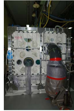
Casaccia – Alfa tight tender for Glove Box dismantling
